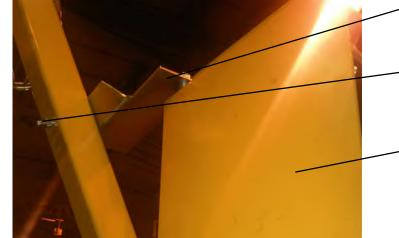
Bolt No 6S03L, Washer Spring No 41S05 and Nut No 9S03
